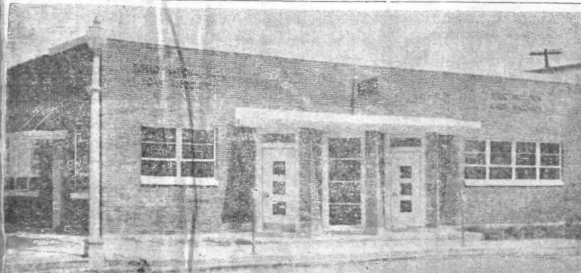
NEW OFFICE BUILDING, south side of which is owned by members of the Tupelo Production Credit Association in 13 counties of NE Miss. Located at 413 South Spring St., Tupelo.
